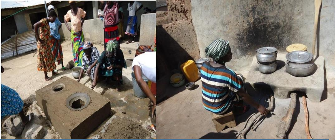
Construction of energy saving mud-stove to reduce quantity of fuel used for preparing house hold food
